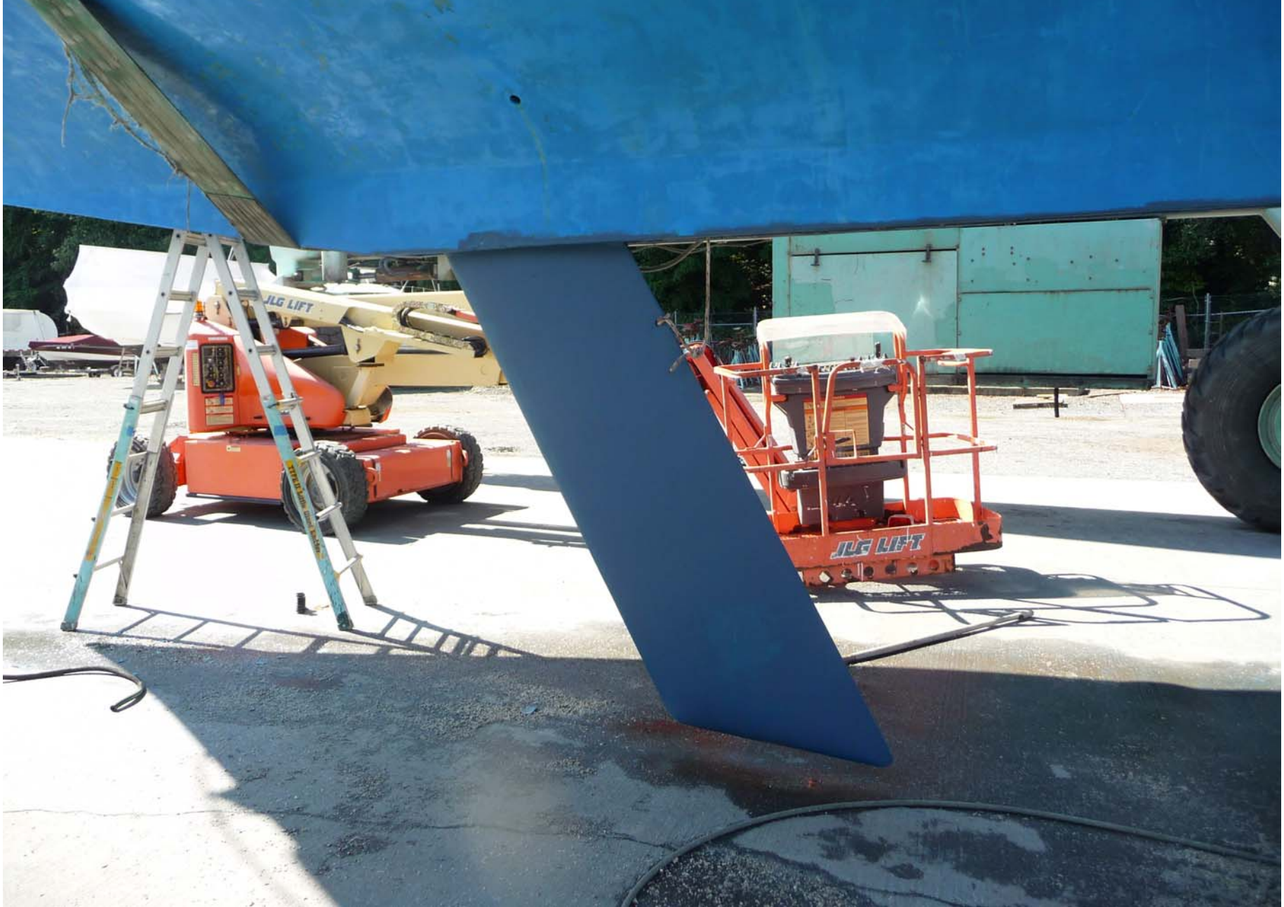
Barnacle free and anti-fouling paint put on.
