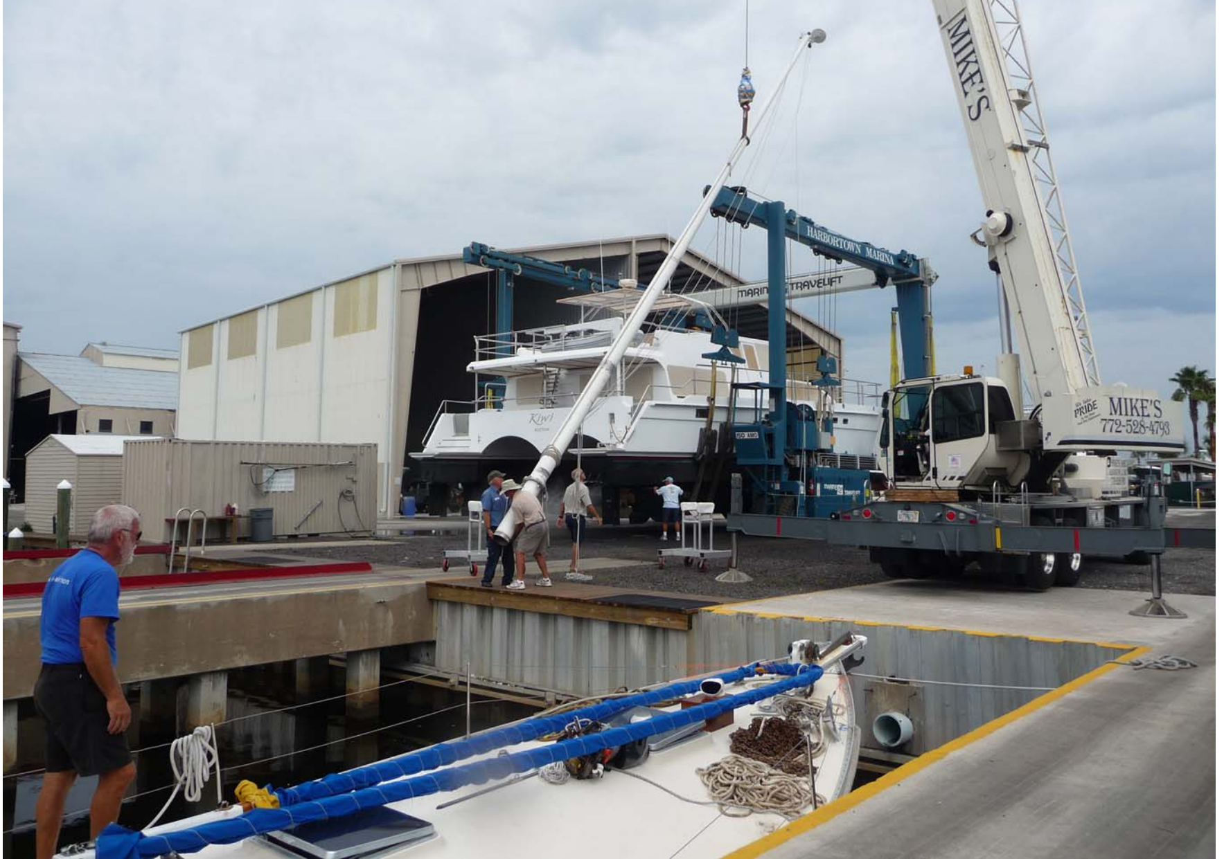
The crane has just lifted out our main mast.
