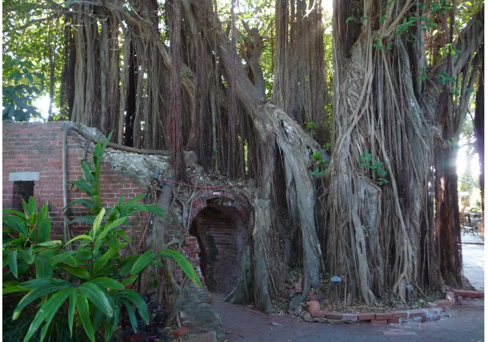
A tree has overgrown the West Martello Tower ruins.
