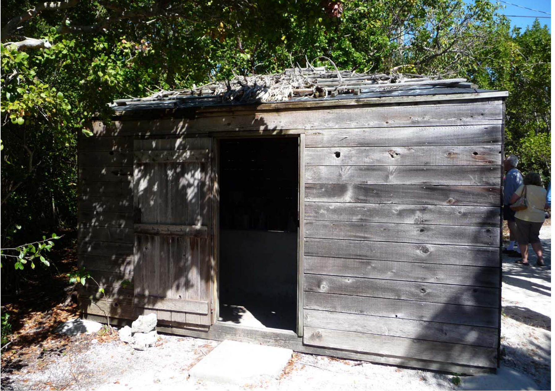
This was the kitchen area.
