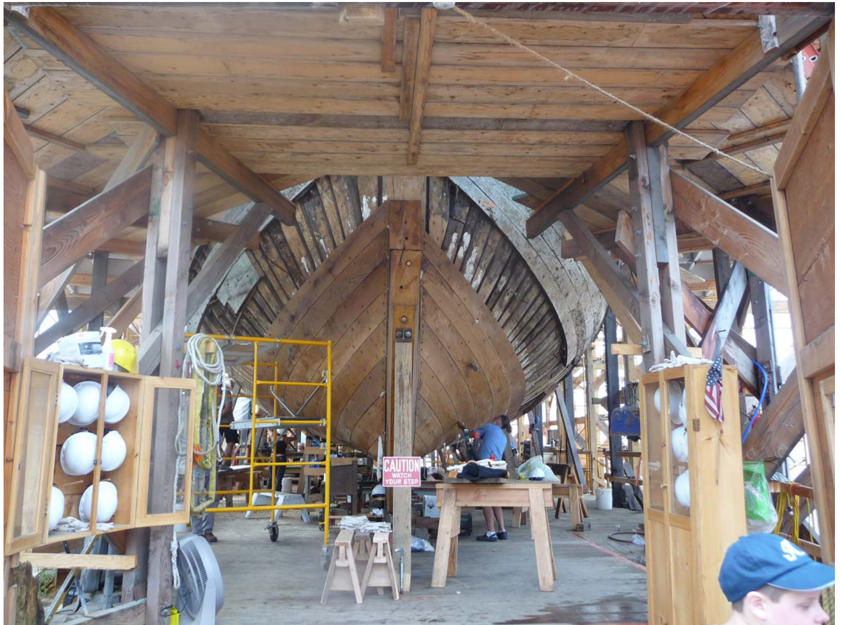
The ongoing restoration of the Charles W. Morgan in the Henry B. duPont Preservation Shipyard.
