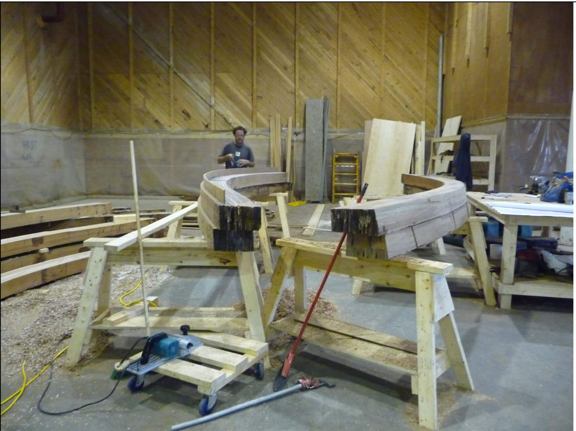
Bluenose II frames get the bevel put on after laminating at Covey Island.
