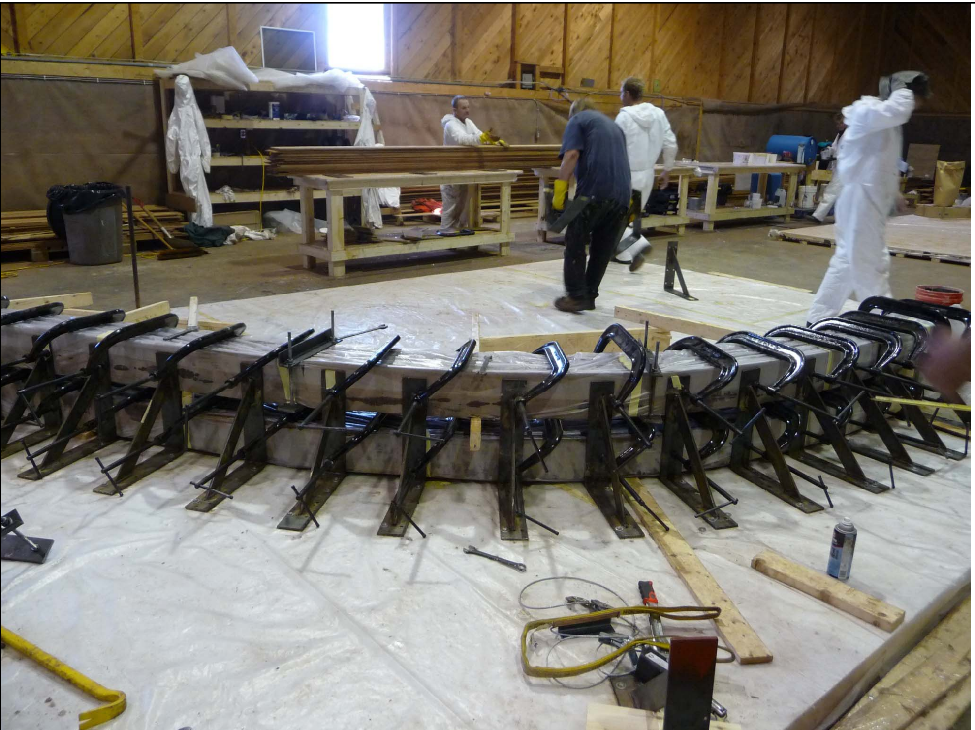
The new Bluenose II frames are laminated together of Angelique wood from Ghana.
