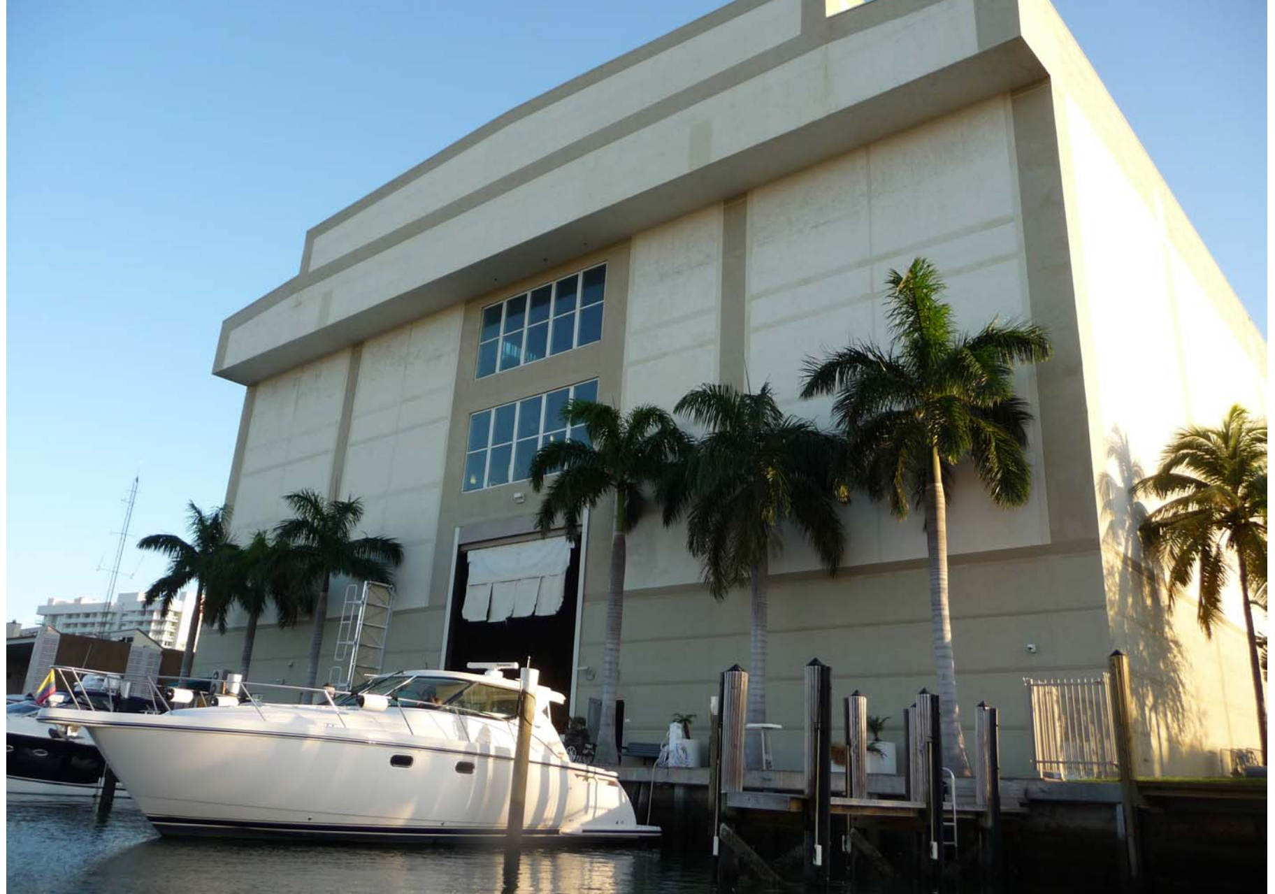
A indoor boat storage building in the 17 th St. canal.
